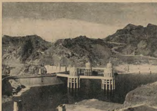
Upper Face of Boulder Dam from Arizona Side
