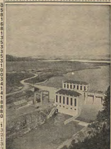
One of Five Power Development Plants on Historic Bear River, Utah
