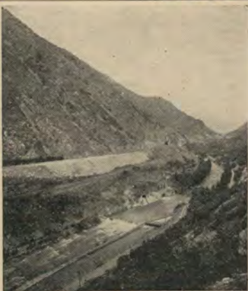
Weber Canyon, Utah, is one of Union Pacific's scenic features en route to California
